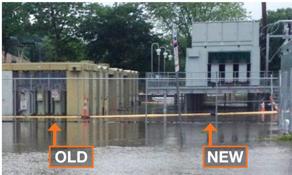
More than 4,600 PSE&G customers in Ewing and Trenton had power at the end of May thanks to Energy Strong. The program built a new, elevated station (on right) that did not flood while the lower old station (on left) flooded on May 27, 2018 after storms. When completed later this year, 490,000 of PSE&G's 2 million customers who lost power during Sandy won't lose power again due to flooding.
