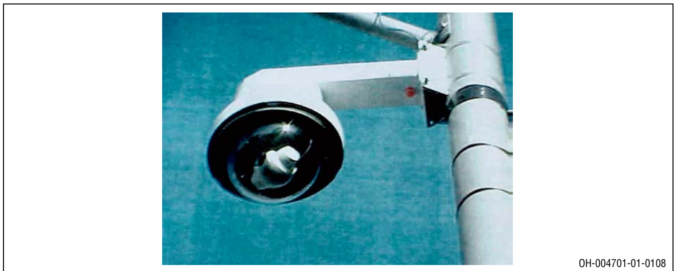
Figure 6.9: Camera Attachment to Metal Pole
