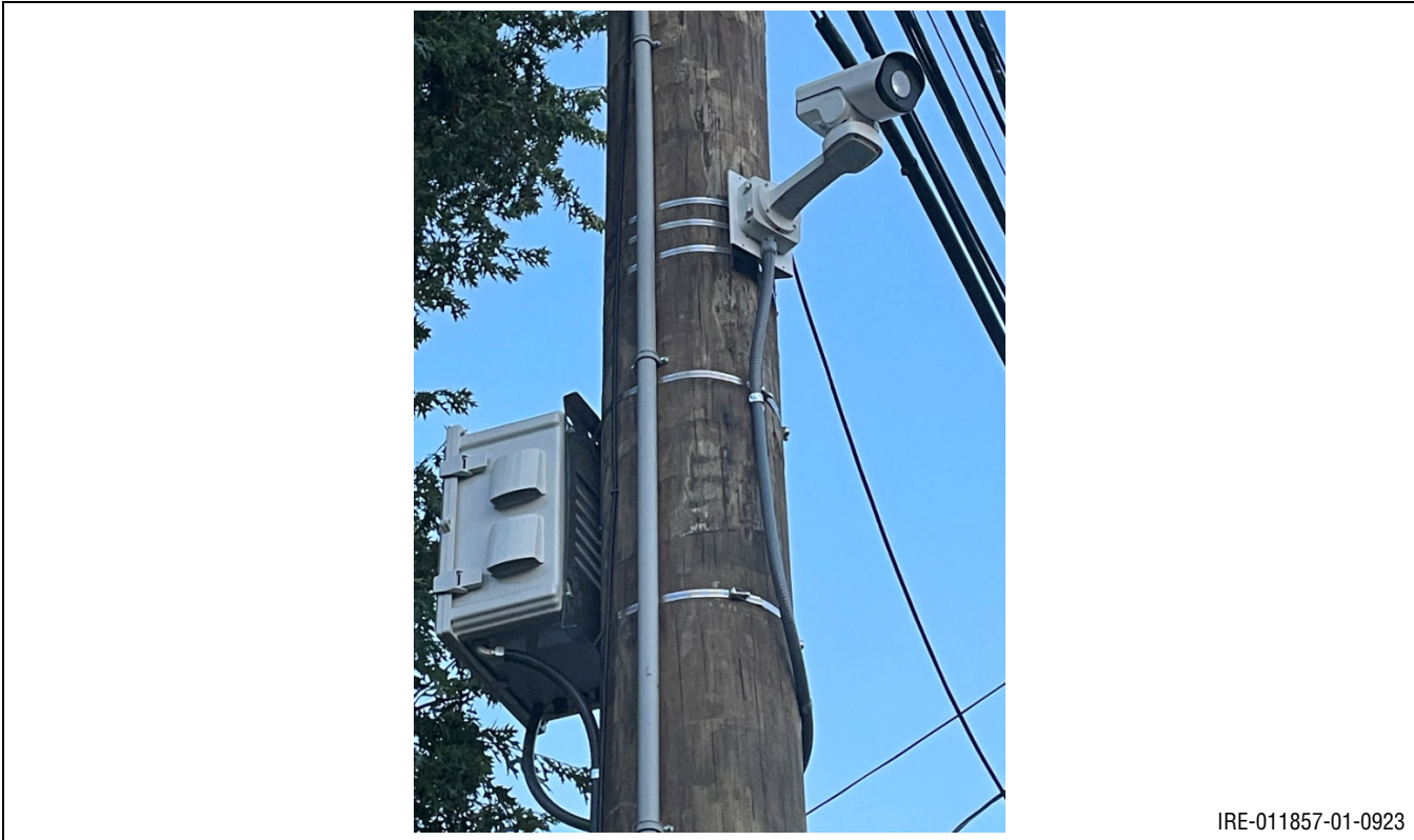
Figure 6.10: Camera Attachment to Wood Pole
