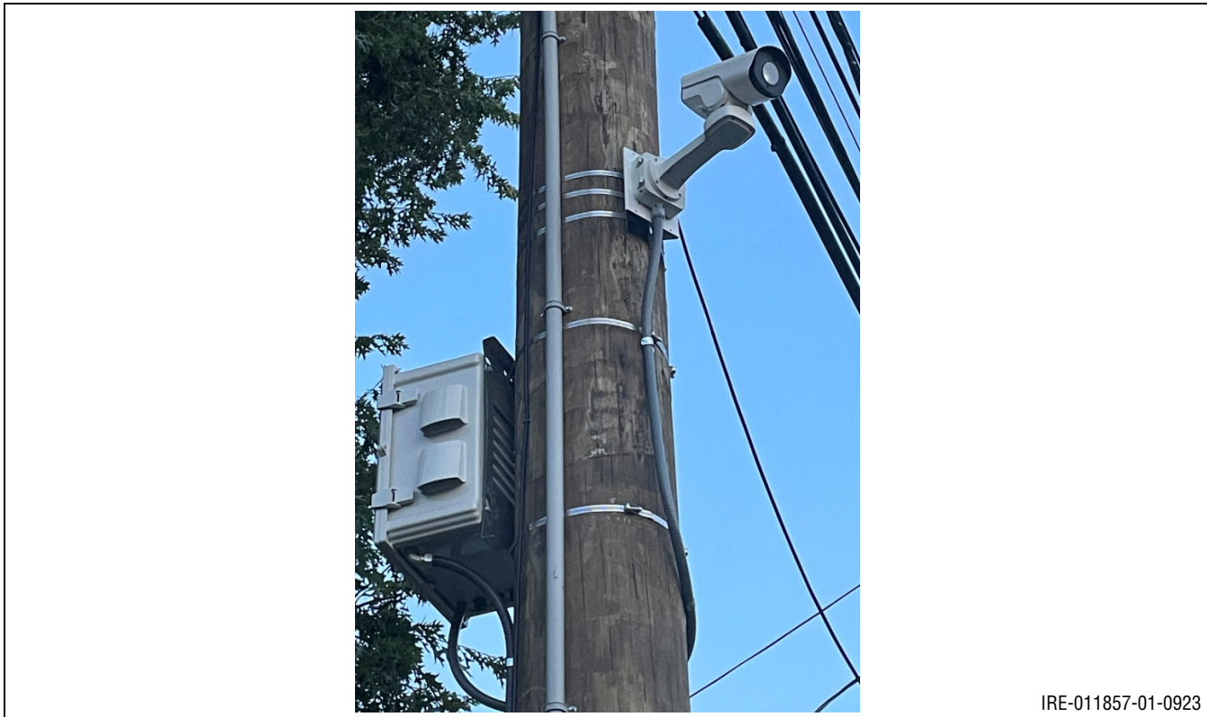
Figure 6.10: Camera Attachment to Wood Pole
