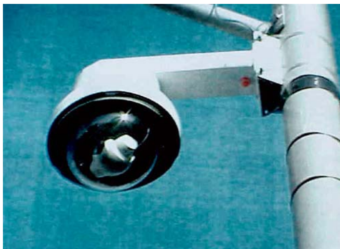
Figure 6.9: Camera Attachment to Metal Pole
