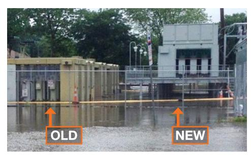
More than 4,600 PSE&G customers in Ewing and Trenton did not lose power in May 2018 thanks to Energy Strong. The program built a new, elevated station (on right) that did not flood while the lower old station (on left) flooded after storms. Now, because of work completed under the Energy Strong Program, 490,000 of PSE&G's 2 million New Jersey customers who lost power during Sandy aren't expected to lose power again due to flooding.
